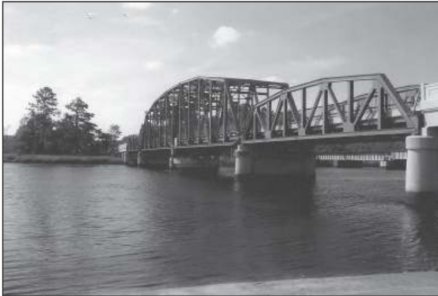
St. Mary's Bridge By Brooke McHaffey
